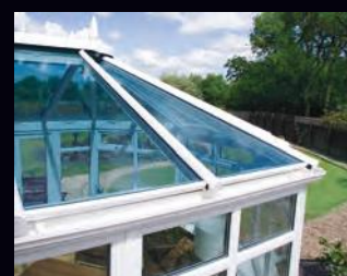
Glass units reduce solar gain in summer & minimise heat loss in winter with treated glass.
